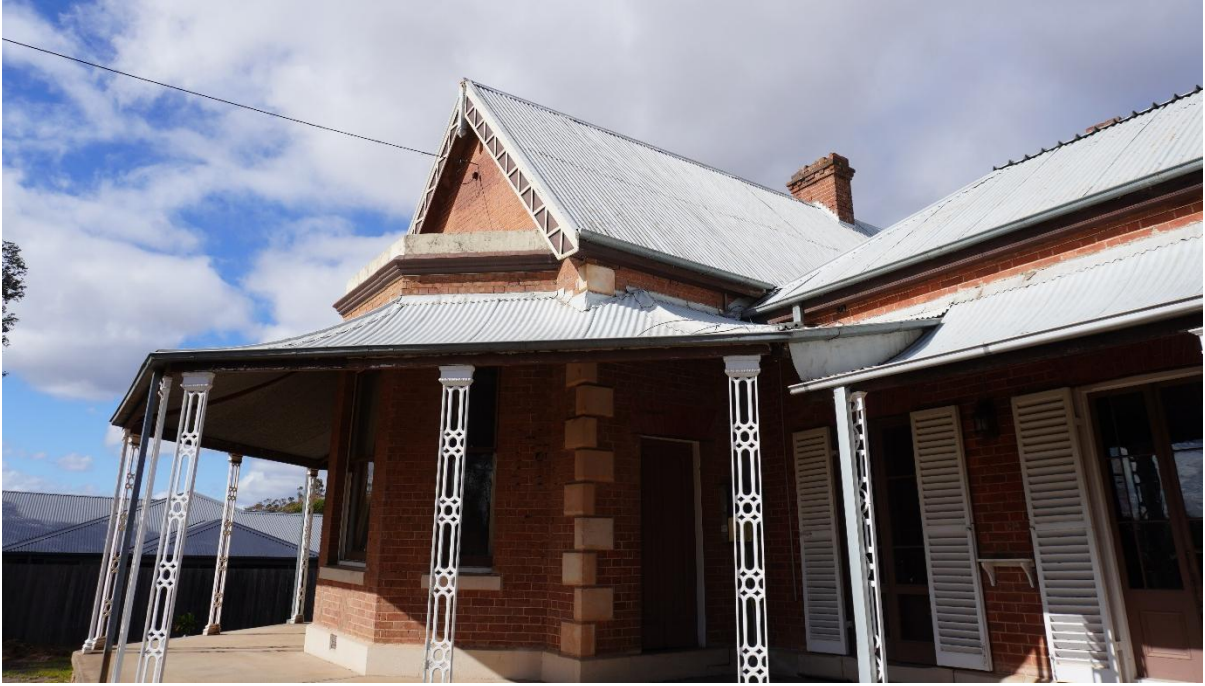
FIGURE 6 FRONT VERANDAH WITH GABLE OVER ADDED. C. LATE 1890S.
