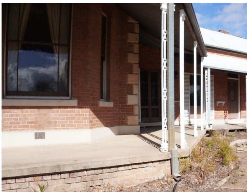
FIGURE 2 CONCRETE PAVED VERANDAH IN THE FOREGROUND AND TIMBER VERANDAH BEHIND.
